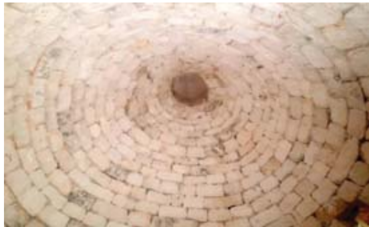
Fig. 1: Alberobello - Bari. Trullo sovrano. Section with masonry and cone structure composition.
