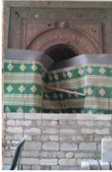
Fig. 5 Left: The method adopted for the Mīhrāb 's protection. Right: The resistance of the built shield. Credits: Dakhel Louay (03 January 2017).
