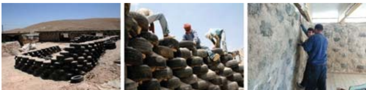
Fig. 5: Left and center, construction phases of the wall structure, http://www.ar-co.org/it . On the right, laying of the clay plaster, https://www.ventoditerra.org .
