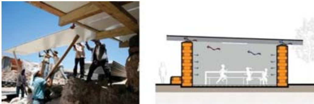
Fig.6: On the left, the installation of the sandwich panels. On the right, cross section with diagram of passive ventilation, http://www.ar-co.org/it .
