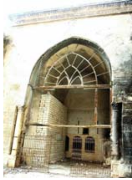
Fig. 5 Left: The method adopted for the Mīhrāb 's protection. Right: The resistance of the built shield. Credits: Dakhel Louay (03 January 2017).
