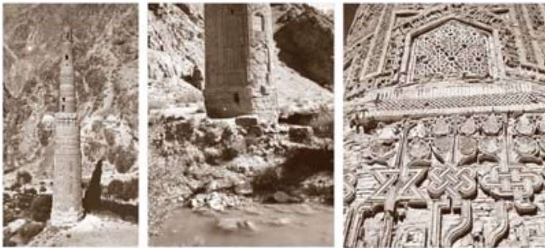
Fig. 01: The Minaret of Jam, erosion caused by the rivers and its decoration. (Photo: © Bruno, 1962).
