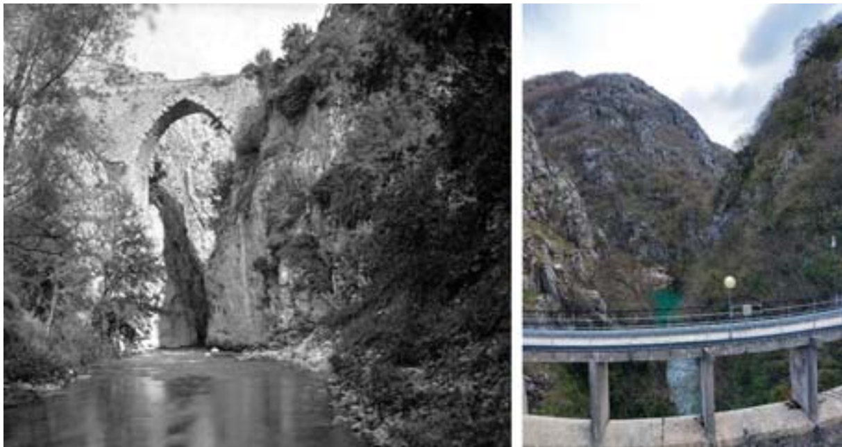
Fig. 5: Ancient bridge with a single ogival arch [14]. Right: spillway of the dam.
