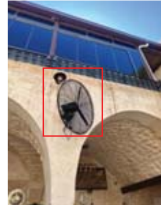
Fig. 12: Hasbahan Guest House & Boutique Otel
