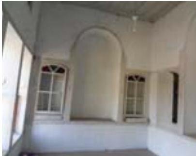
a. Nahrin Otel/ Before restoration
