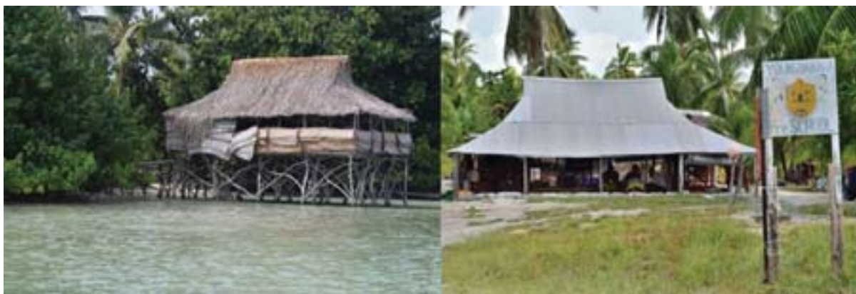
Fig. 3: Left: the roof of a traditional house made with pandanus leaves. Right: example of a galvanized sheet roofing.
