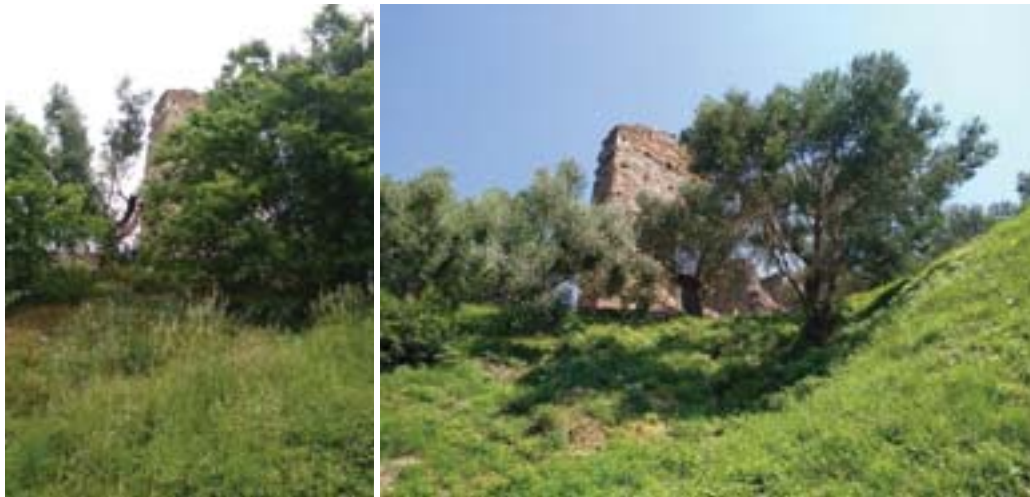
Fig. 6: View of the large pylon before and after the 2020 interventions.
