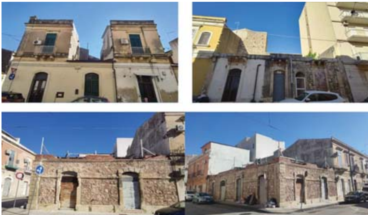
Fig. 2: discontinuity in the façades
