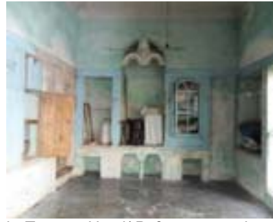
b. Tessera Hotel/ Before restoration
