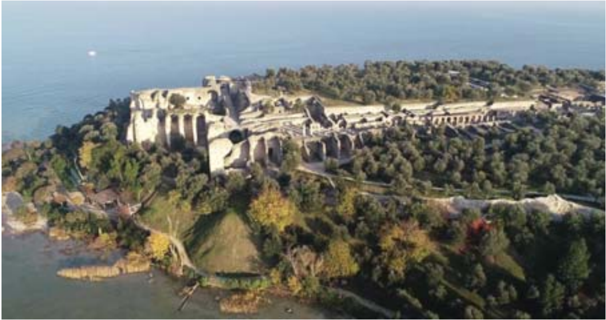
Fig. 1: Aerial view of the Western side of the Grotte di Catullo.
