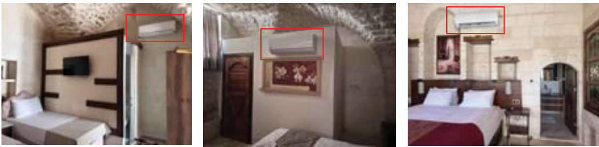
a. Hasbahan Guest House & Butik Otel b. Müzepotamia Guest House c. Tessera Hotel Fig. 20: Air conditioners added inside the rooms
