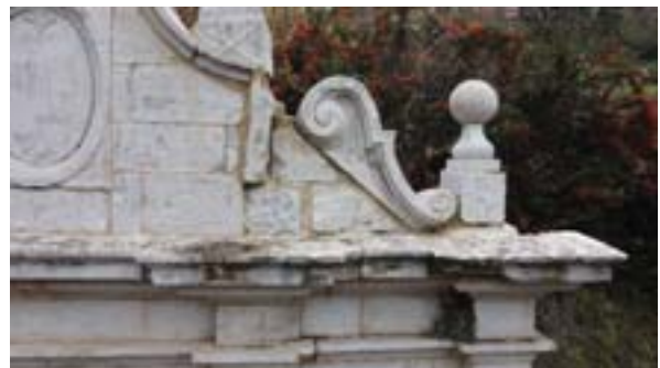
Fig. 7: Photo of part of the top of the Fontana dei Ciechi; part of the missing moulding is shown in the foreground.
