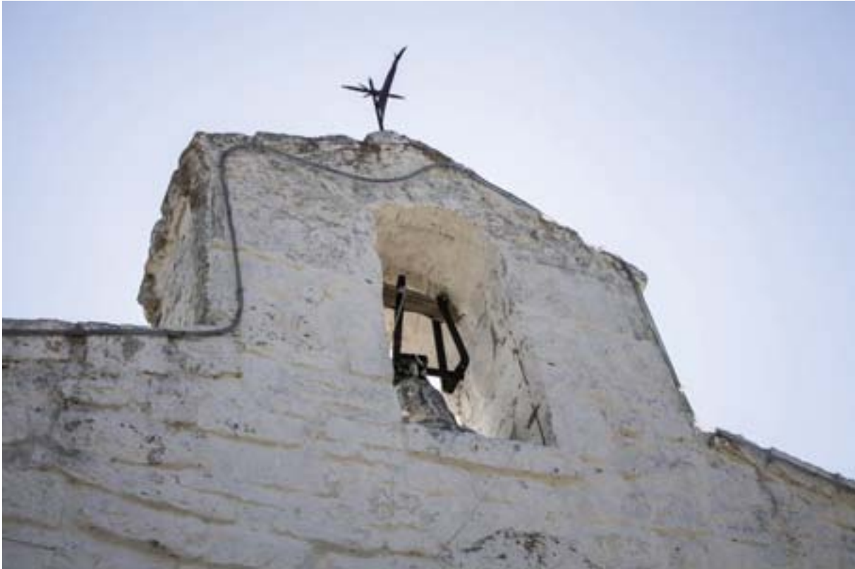
Fig. 3: Photographic survey. Detail of the bell gable on the main elevation
