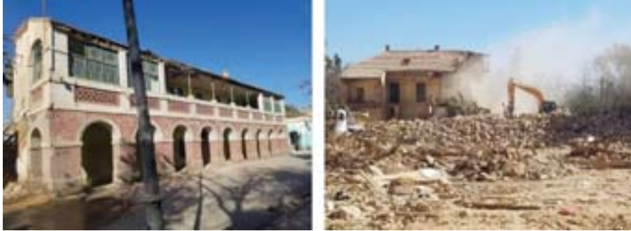
Figure 4. Demolition of the Sahara Hotel in 2023 [16].
