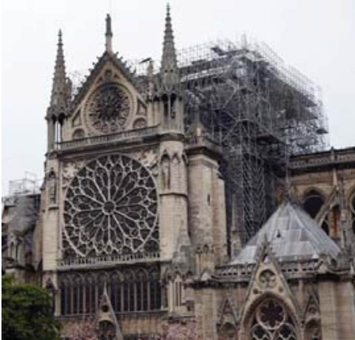
Figure 2. Cathedral restoration process after the fire in 2019.
