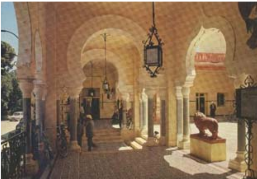
Figure 18. View of the entrance portico of Biskra city hall. On the right, the lion statues after shifting [59].
