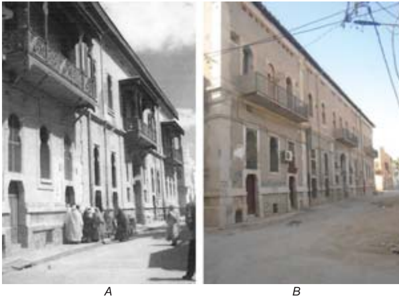
Figure 2. The rear façade of Biskra city hall: A) Old postcards showing the wooden balconies [14]; B) Current view showing the transformation of the wooden balconies.
