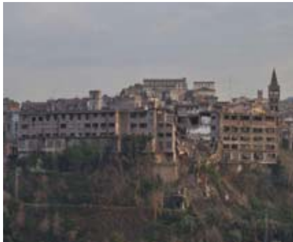
Figure 4. Present day situation (2020): result of the massive collapse of 2009 on a section of road, "Via degli Stabilimenti", that runs through a tunnel (Source: Municipality of Tivoli).
