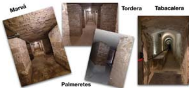
Figure 9. Four of the shelters rehabilitated in the DUSI Project
