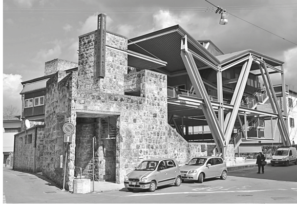
ID 016 Structure/external envelope relationship in the Monte dei Paschi di Siena headquarters in Colle Val d'Elsa (SI) by Giovanni Michelucci
